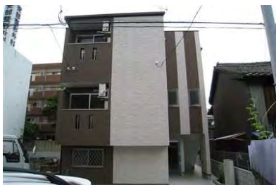
CAMELOT HAKATA canalside (7月竣工/6戸：福岡市博多区)
